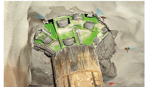
Breakthrough of reaming head.
