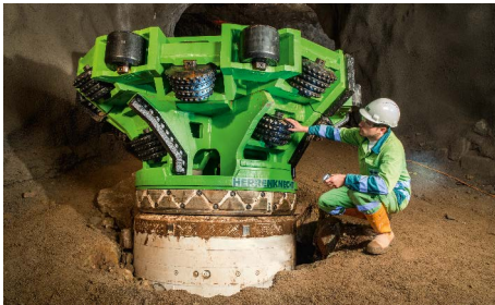
Reaming head on boring unit before collaring.
